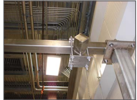
Above: Detailed view of the crane suspension
